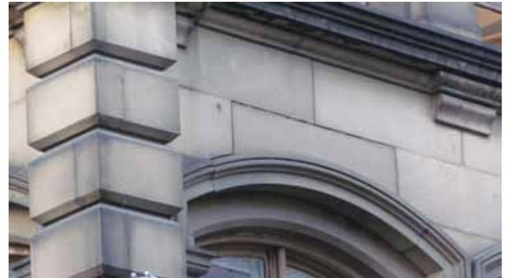
**38 GREENE STONE FACADE** - After low pressure water cleaning and Sure Klean application
