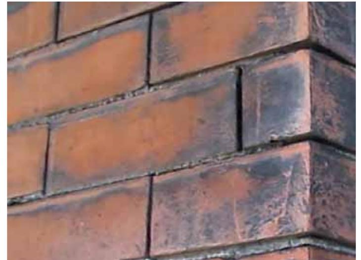
**38 GREENE MASONRY FACADE** - After low pressure water cleaning and Sure Klean application
